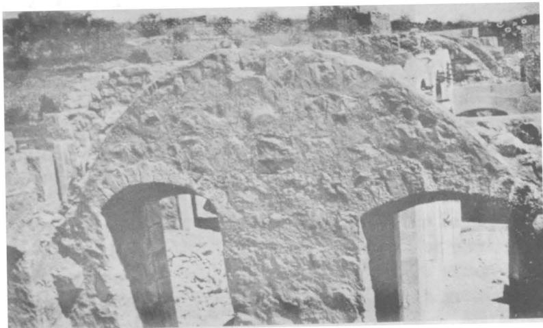
Fig. 1. One crescent shaped wall of a house in process of construction. The first protruding stone of the *rukbeh*, the *zifr*, is seen in the left corner. On the top of the *hlāl* the niche into which a beam of the *tūbār* comes to rest is visible.
