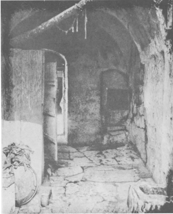
Fig. 1. A cistern built under a house, and opening in a room of the lower story.
