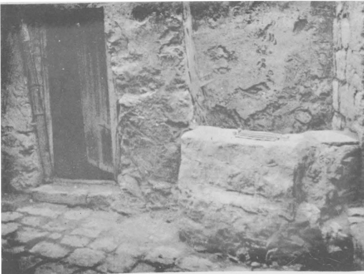
Fig. 2. A cistern in the court of a peasant's house.
